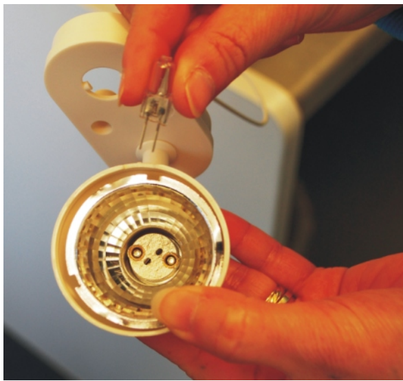
Removal of Tungsten Halogen Bi Pin
